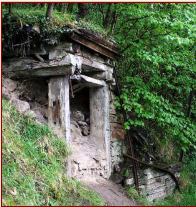
A disused rail siding at Long Meg Gypsum Mine
